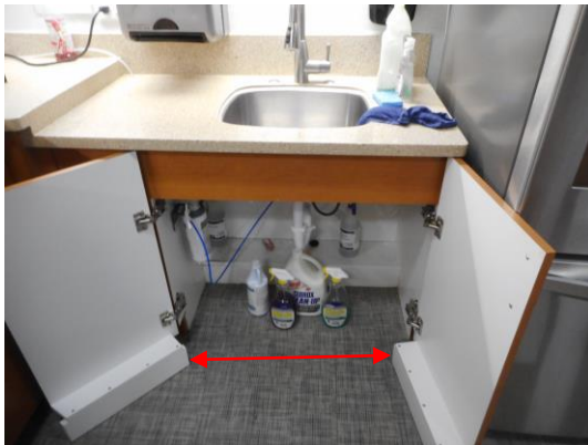
Photo 10: A sink with a forward approach is provided in the employee break room (a parallel approach is not possible due to the depth of the adjacent refrigerator). This is a good example of accessibility. The width of the clear floor space is only 29" (vs. 30" minimum) due to the toe kick detail.
