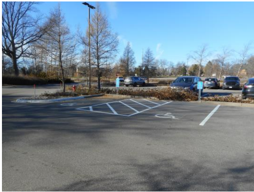
Photo 1: Accessible parking spaces have been designated near the main entry. This is a good example of accessibility. Additional recommendations include raising the signs to 60"-66" (measured to the bottom of the sign above the parking surface); currently at 33".
