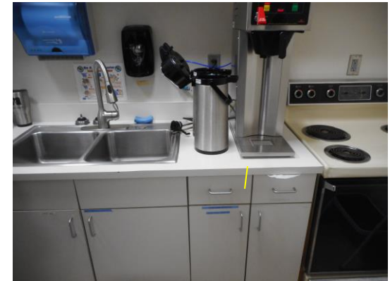
Photo 12: A full kitchen (including a range) is currently provided on 2 nd floor. There are currently no features of accessibility provided within the kitchen. Note- if the range were eliminated there would be fewer accessibility requirements for the kitchenette such as no accessible work surface requirement and a parallel approach would be allowed at the sink.
