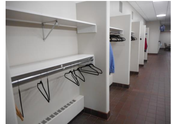
Photo 6: The coat closet area near the main entry includes an accessible hanging section. This is a good example of accessibility.
