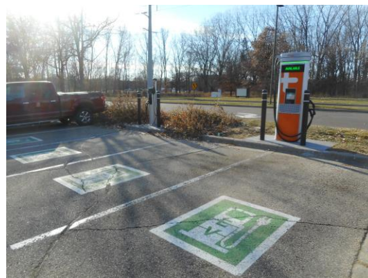
Photo 17: There are currently 4 EV charging spaces located along the west perimeter of the parking lot (2 different style charging stations). There is not currently an accessible route to the charging station and none of the spaces currently has an adjacent aisle.
