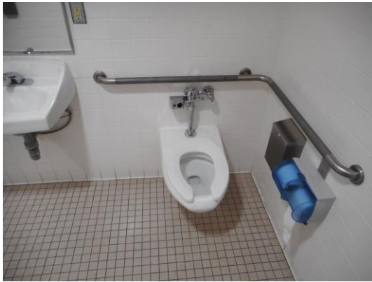
Photo 13: A single-user toilet room is provided on 1 st floor adjacent to the elevator. This room provides many features of accessibility, but does not fully comply with current requirements at this time. Additional modifications include replacing the grab bars and relocating the lavatory to outside the toilet clearance.
