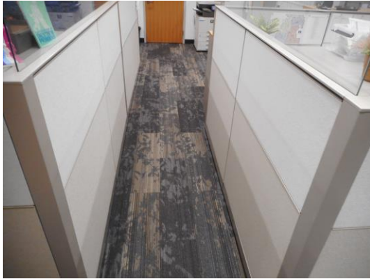
Photo 13: The distance between the cubicle partitions within the Administration office is 35" (vs. 36" minimum).
