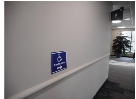
Photo 15: Near the 2 nd floor toilet rooms signs directing to accessible toilet rooms have been posted. The signs are directing to the toilet rooms located in City Hall. Additional details could be included to provide users more information about the location of the toilet rooms as well as directing to the 1 st floor single-user toilet room.
