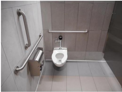
Photo 7: The multi-fixture toilet rooms on both levels have been remodeled and features of accessibility were incorporated. This is a good example of accessibility.
