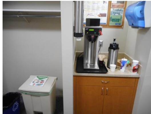
Photo 11: A coffee station is provided in passage 151 (outside Minnetonka Mills). Currently most elements are above the maximum reach of 48" AFF, including: coat rack, towel dispenser (at 61 1/2"), cup dispenser (at 54") and hot water dispenser (at 58").
