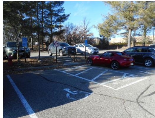
Photo 2: There are 2 parking spaces designated that face west; the aisle aligns with stairs from the upper portion of the parking area. These spaces are not located on the shortest accessible route to the main entry.
